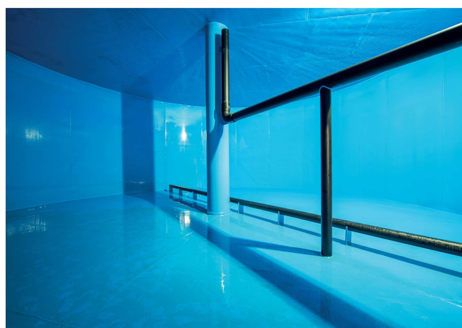
POTABLE WATER TANK-LINING
