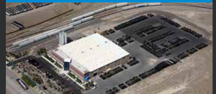
AGRU NEVADA FERNLEY, NV/USA
