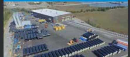
XXL PIPE PRODUCTION FACILITY CHARLESTON, SC/USA
