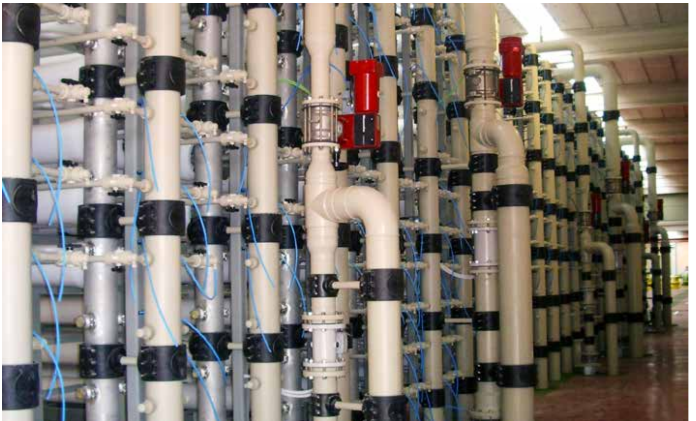
AGRUCHEM piping systems made of PP meet the high purity requirements essential for reverse osmosis.
