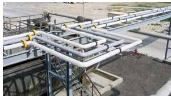
Figure C.6: U-shaped expansion bend
