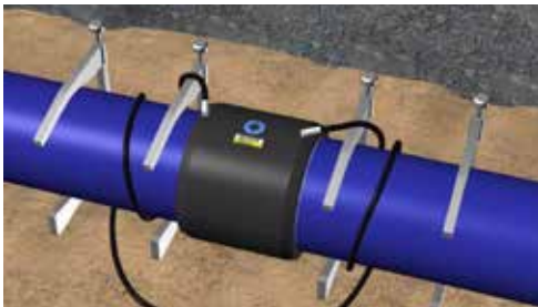
Figure D.21: Connecting the welding machine
