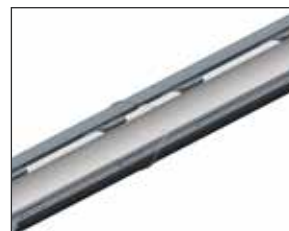
Figure A.17: Welding of the outside pipe
